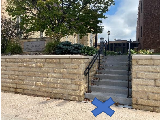
Stairs by St. Michael Church
